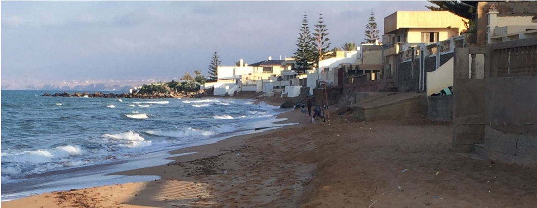
Figure 2: Ocean dangerously close to homes in Nador (Photo credit: Muller, 2016)
